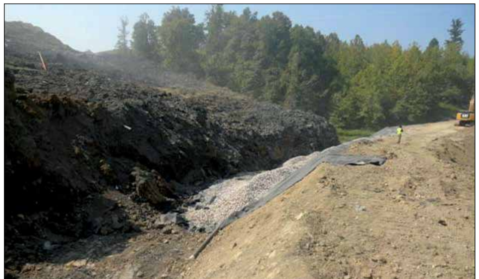
TOP: Big Run Landfill in spring 2013 before the slide. DWM photo ABOVE: Immediately following the slide, a large wall of garbage (left) towers above facility personnel in the yellow vest. Photo by Rodney Maze
